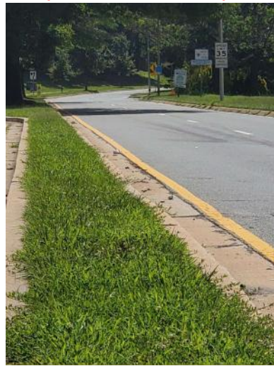
Approaching North Entrance - Heading East 500' Away
