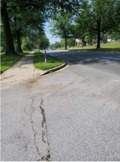
At West Entrance Looking Left/South
