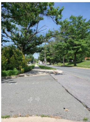
At North Entrance Looking Left/West
