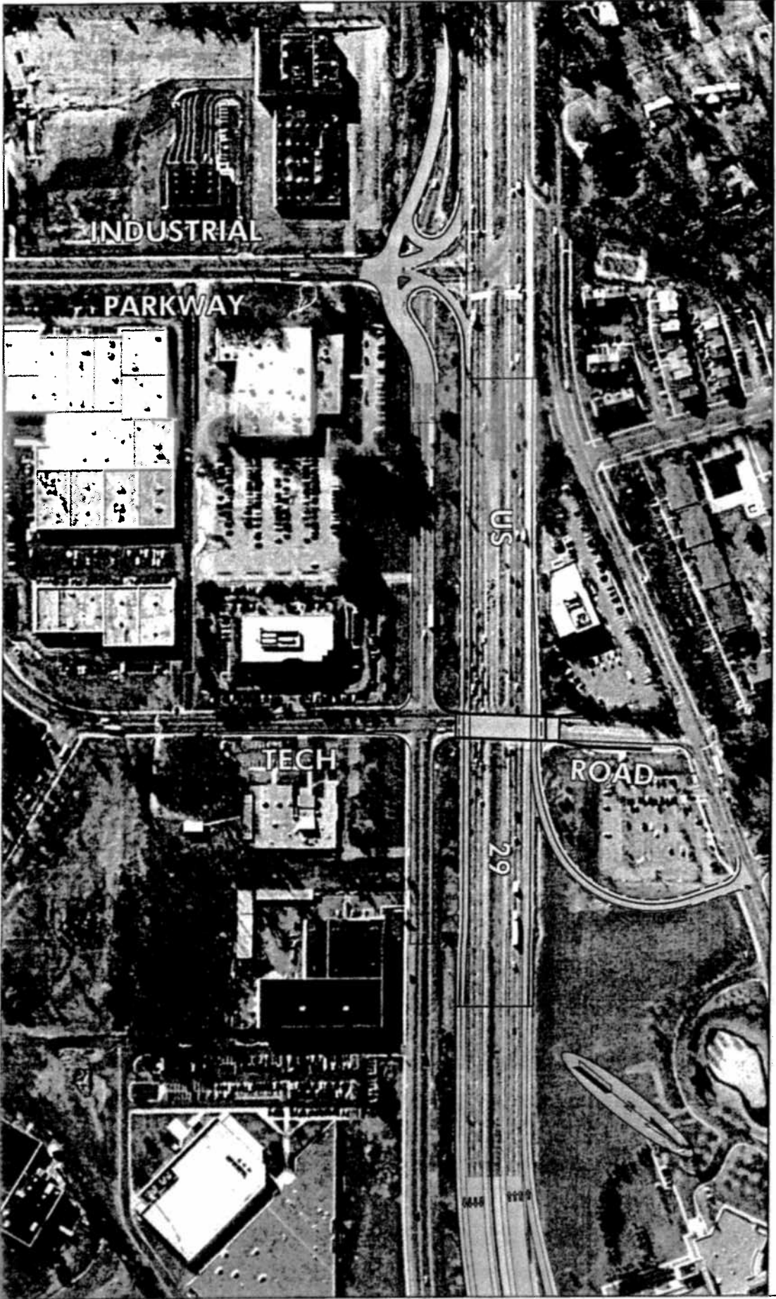
US 29 at Tech Road / Industrial Road
